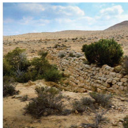
Rock terraces have been built across the wadis to capture runoff and to generate gradual deposition of soil. ©SG
