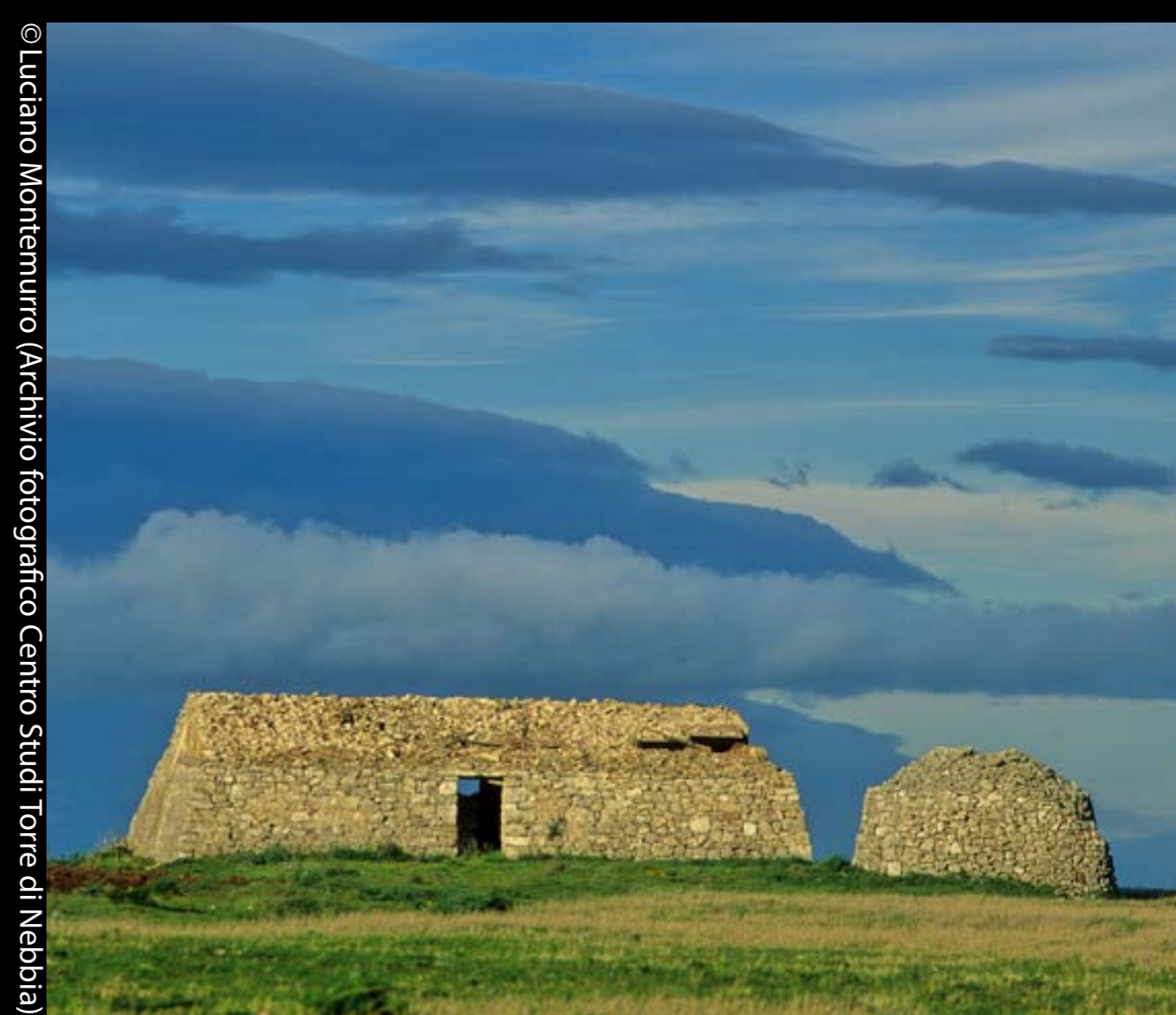
Now abandoned buildings, formerly used by shepherds practicing transhumance.
