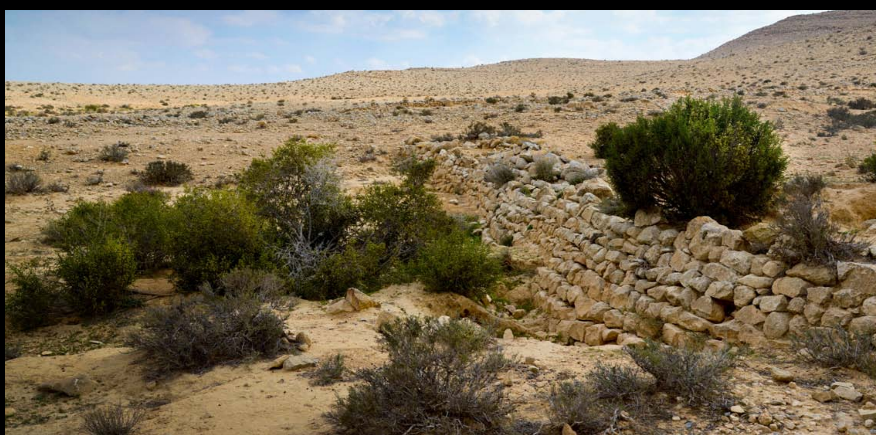
Rock terraces have been built across the wadis to capture runoff and to generate gradual deposition of soil.
